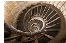
The 311 step stairwell
